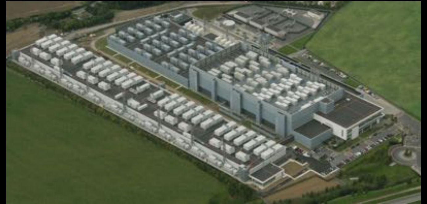
15,000sqm, 16MW single storey Data Center (Argo's CTE Leader worked on this project while working for RKD)
