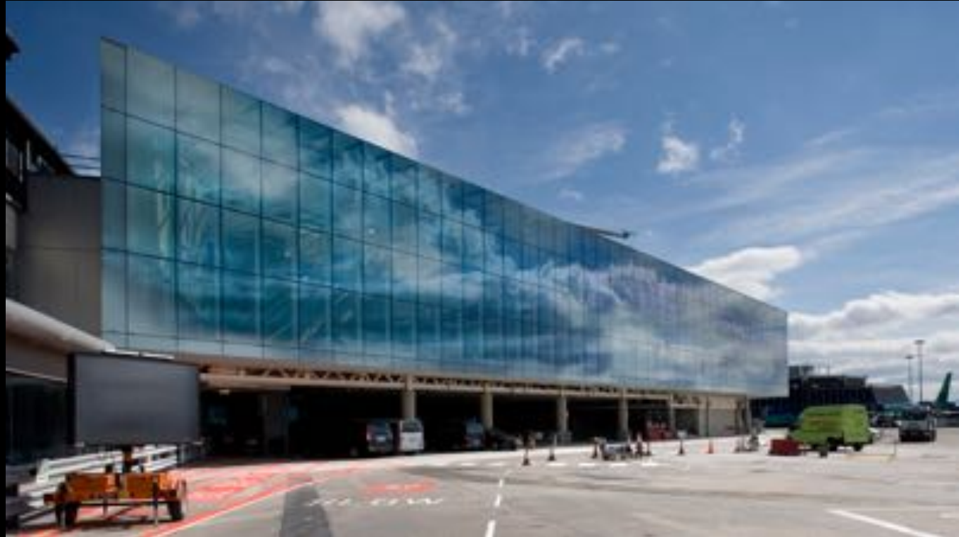
Dublin Airport Terminal One Extension – Dublin, Ireland
